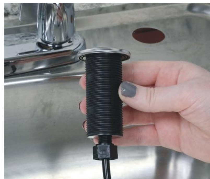
Remove Nut & Washer & Connect Hose
