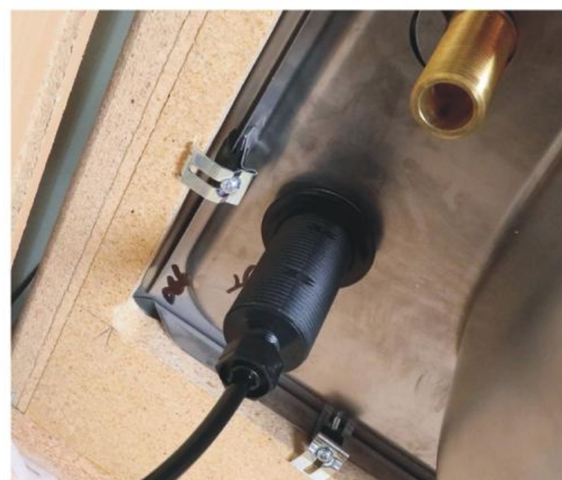
Thread Nut & Washer onto Assembly
